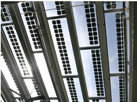
*A building integrated solar photovoltaic (BIPV) system installed in the skylights at the Marjorie McNeely Conservatory at Como Park in St. Paul, Minnesota.*
